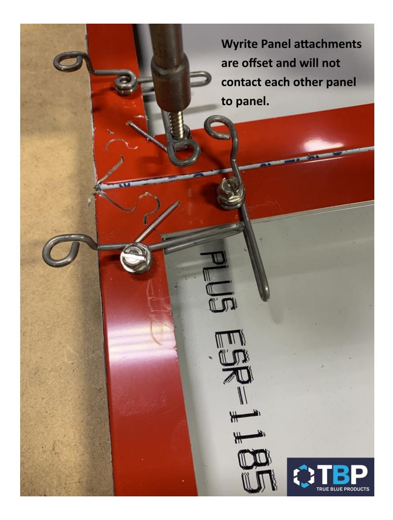
Wyrite Panel attachments are then fastened on the top and bottom of the panel to horizontal girts, or on the left and right sides to vertical girts, fastened perpendicular to stiffeners (along the long sides of the panels). The attachments on the sides that are not fastened utilize the Wyrite attachments only to support reveals. Outside corners on buildings may require all 4 sides to be fastened to account for wind wrap.
